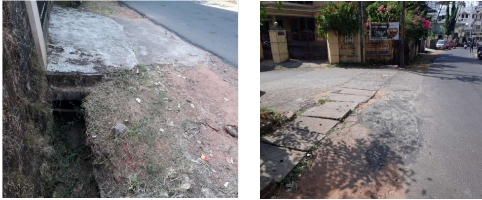
Figure 38 Existing drains along 19-BR Karkera Road
