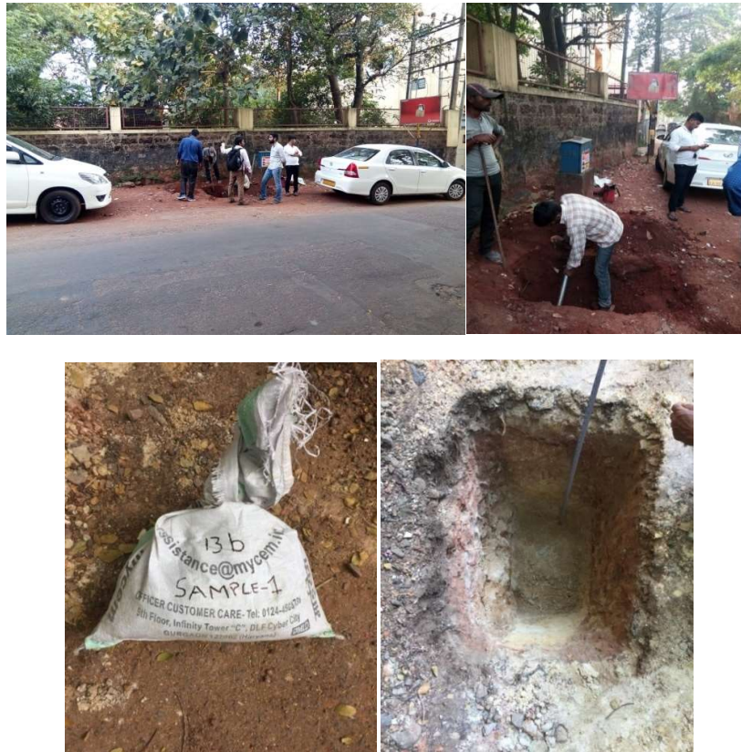
Figure 19 Trial Pits Survey Site Photographs Traffic Surveys and Analysis
