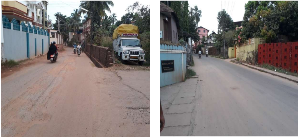
Figure 41 Existing drain along Road 23
