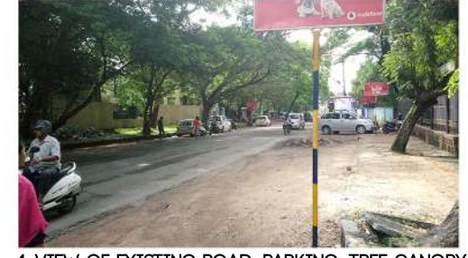
4. VIEW OF EXISTING ROAD, PARKING, TREE CANOPY AND SIGN POLES NEAR KADRI PARK
