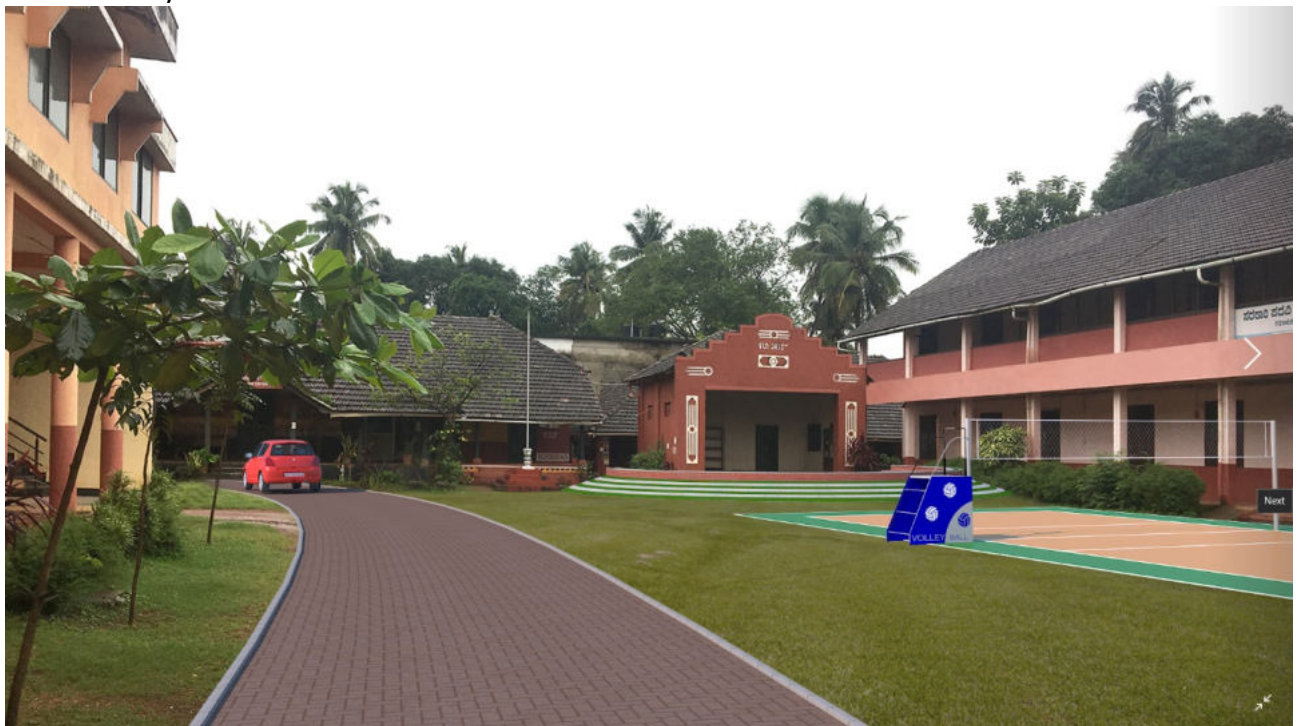
After- Entry Side
