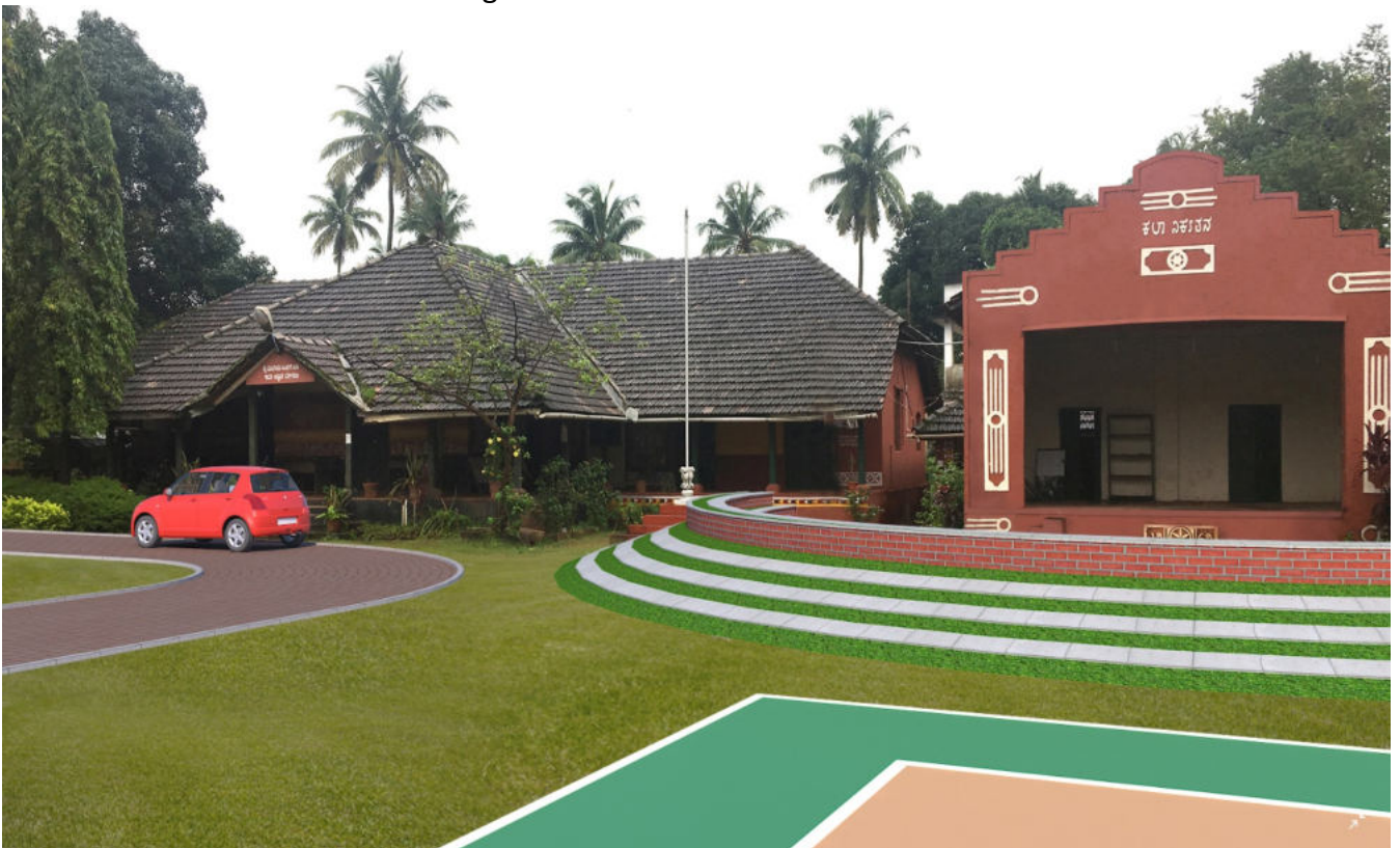
After- Front of Admin Block & Stage
