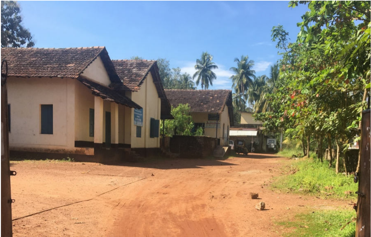
Before- Entrance Path
