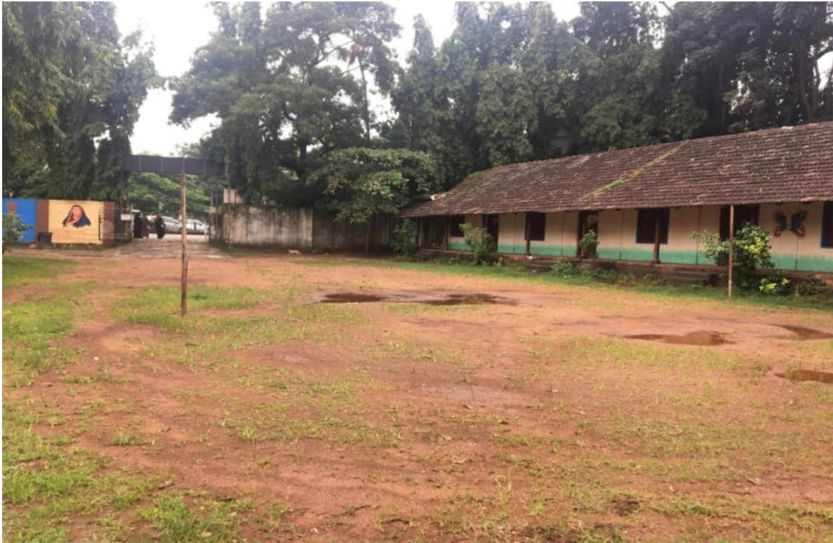
Before- Main Entrance & Ground (From Inside)
