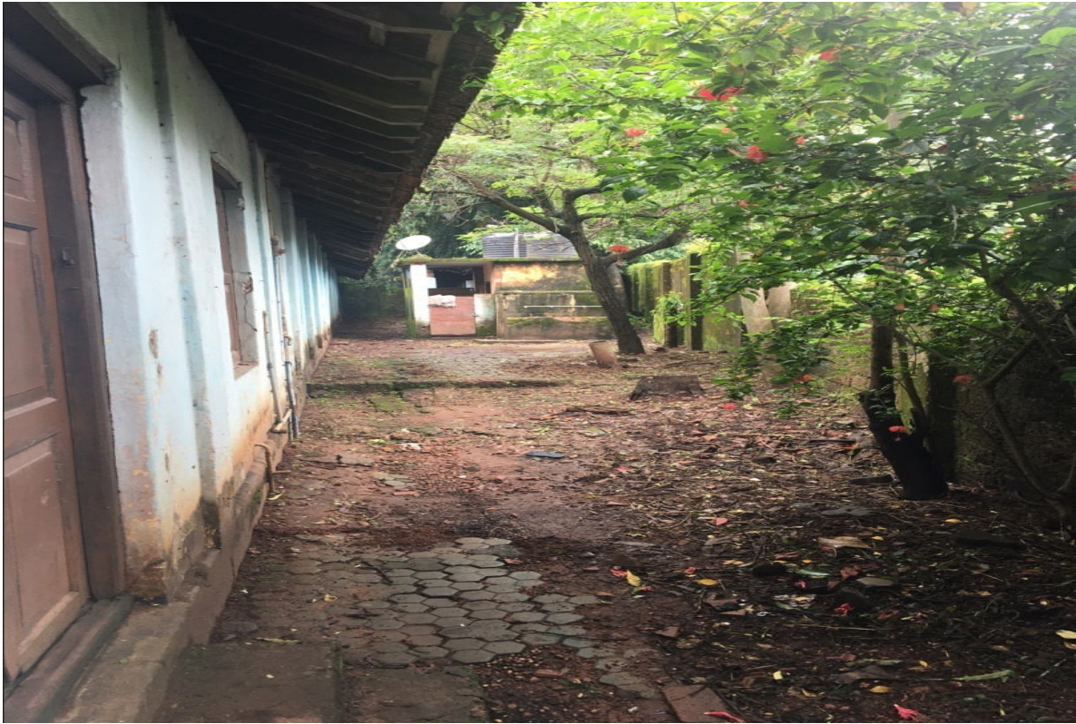
Before- Backside of Building
