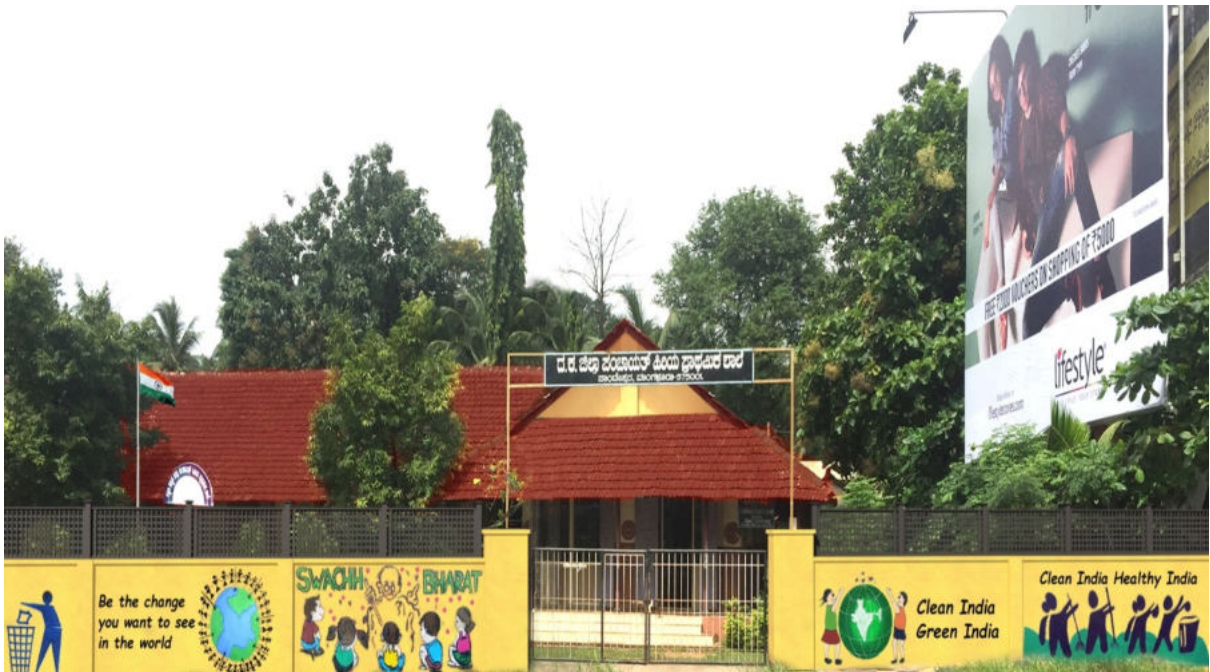
After- Main Entrance
