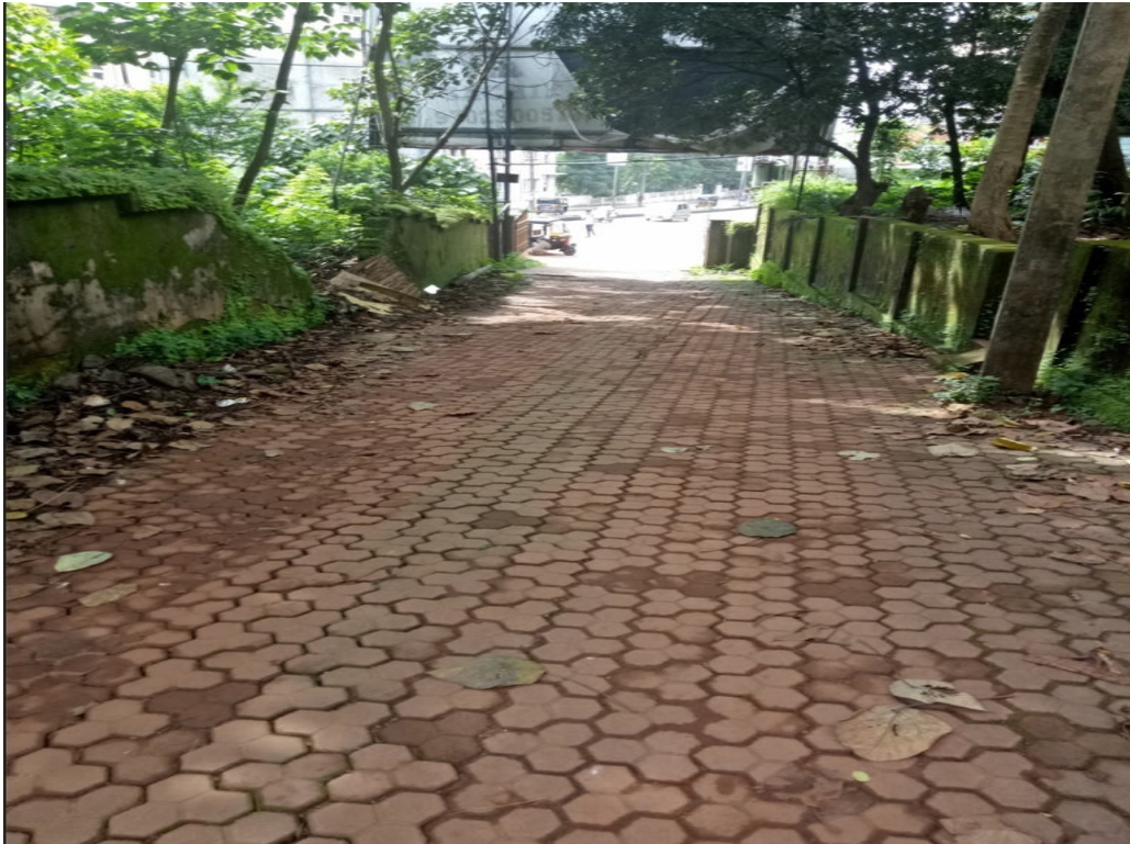
Before- Entry Ramp
