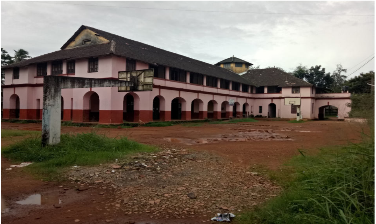
Before- Basketball Court
