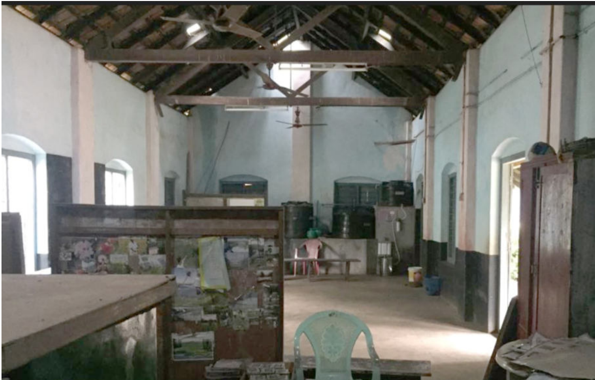
Before- Inside Classroom
