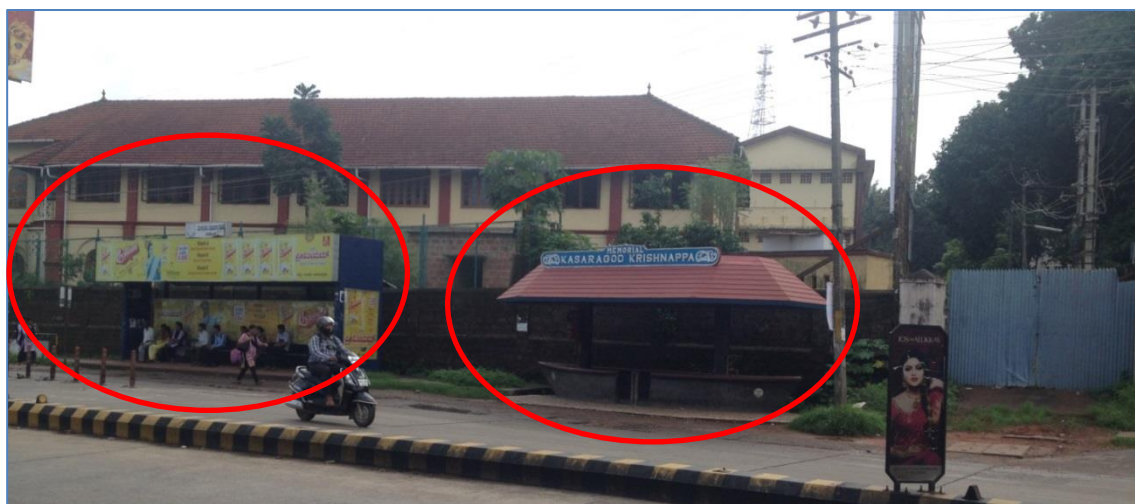
Figure 3: Existing Bus Shelters
