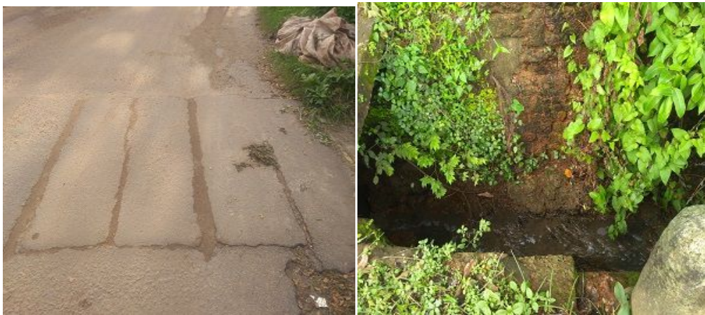
Figure 10 Drains in Good shed Road
