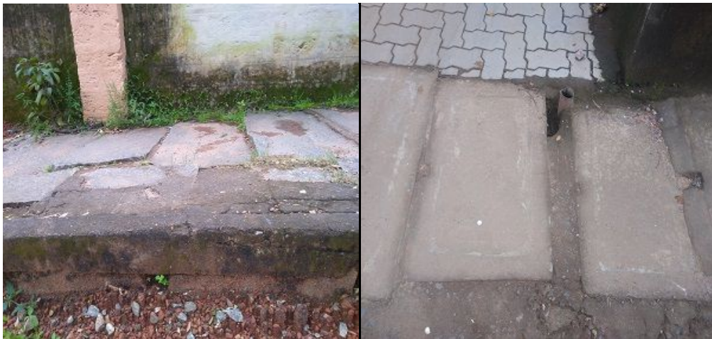
Figure 9 Existing drain in good condition along Rosario Road
