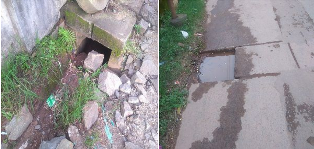
Figure 8 Existing cross drain and Drain in damaged condition along Rosario Road
