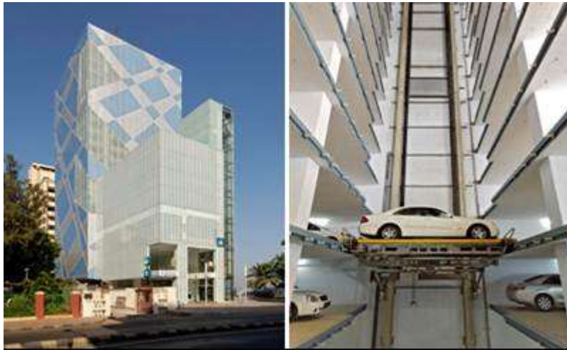
View of Automated parking system installed by Wöhr Automatik Park Systeme, GmbH at Akruiti Skypark in Mumbai
