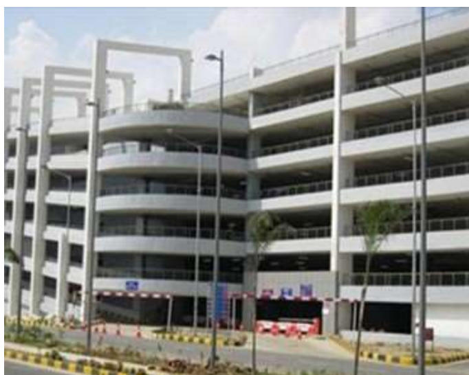
View of Ramp based MLCP at Delhi International Airport
