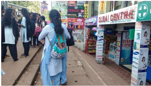
Drain present at the lower level than the road level
