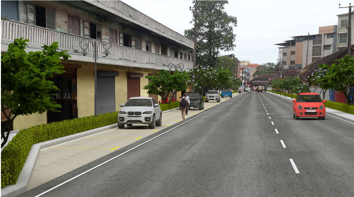
Nellikai Road : After
