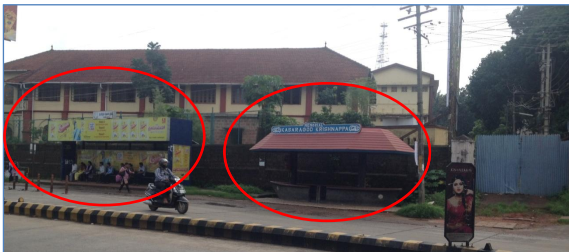
Figure 3: Existing Bus Shelters
