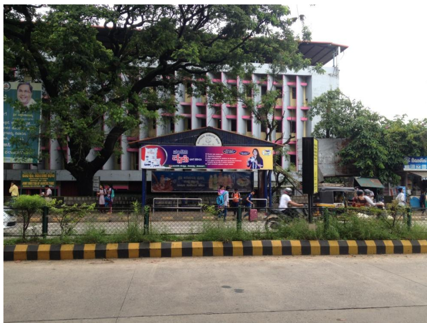
Figure 5: Existing Bus Shelter Design
