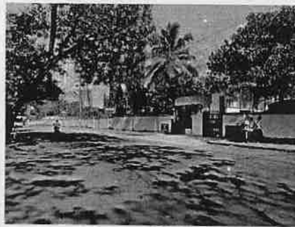
4B. VIEW OF ENTRANCE GATE OF AKASHWANI KENDRA - as seen from Kadri Park Musical Fountain side
