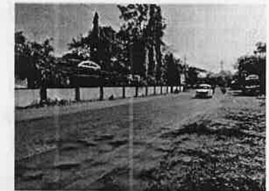
4. VIEW OF BALA BHAVANA- as seen from Shri Jogi Mutt compound
