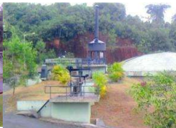
Primary Treatment Unit
