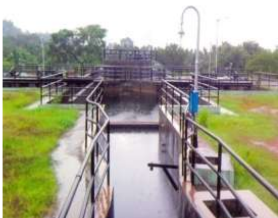
Primary Treatment Unit
