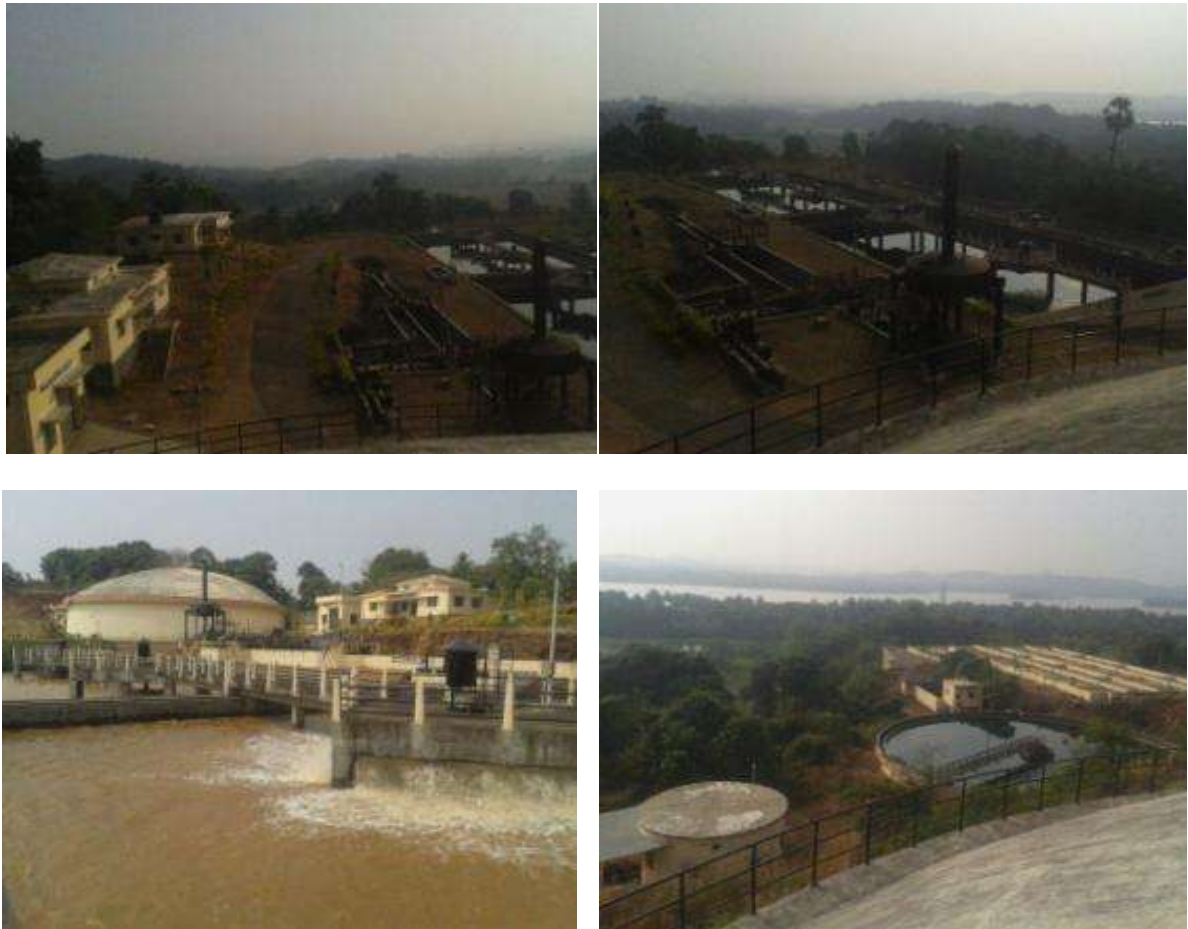
Figure 2-5 20 MLD STP at Bajal
