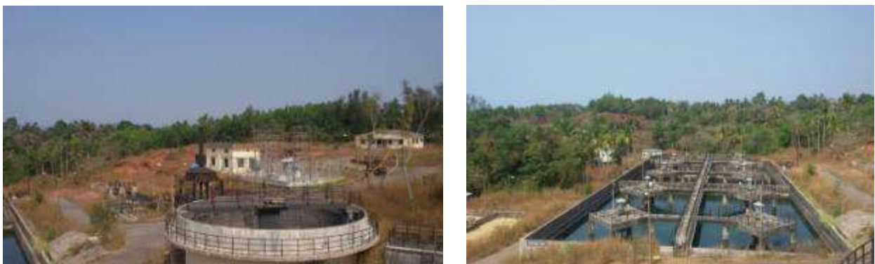
Figure 2-6 16.5 MLD STP at Suratkal
