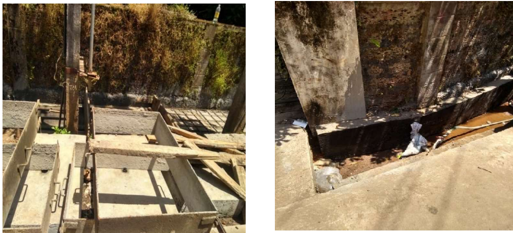
Figure 40 New drains being constructed along Road-10
