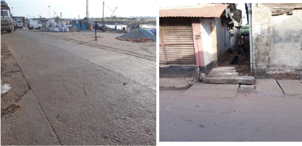
Figure 44 Existing drain along Road 20 & No drain along Port area
