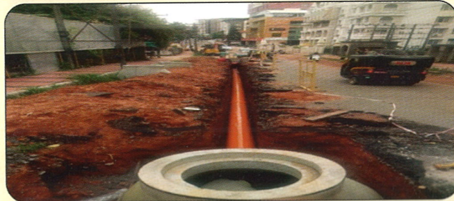
Total project cost : Rs. 42.5 Crores. (5 packages)
