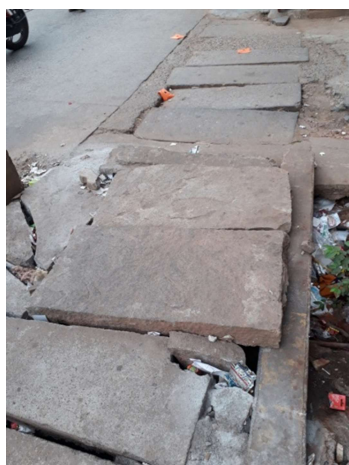
Existing discontinuous drain along Road-13b
