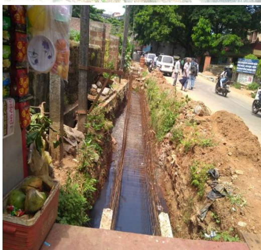
Existing drain and newly constructed drain along Road 7d
