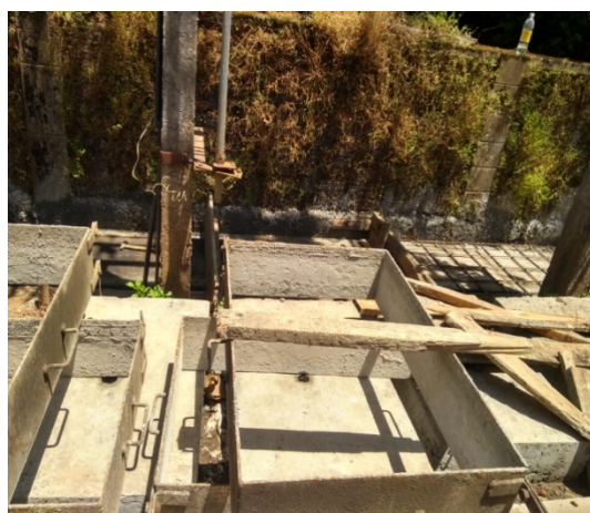
New drains being constructed along Road-10
