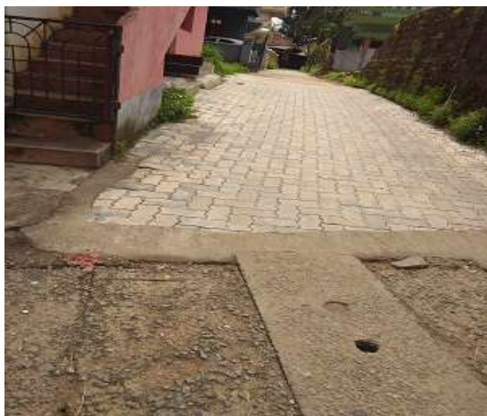
Interlock Pavements in Zone-6
