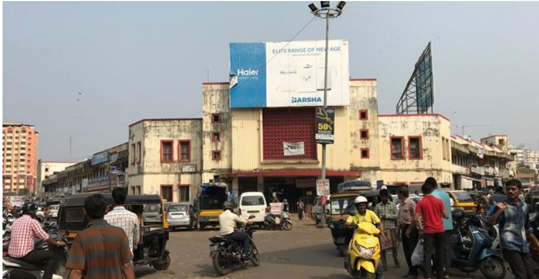
Figure 3 Front Elevation and Main Entrance of Central Market
