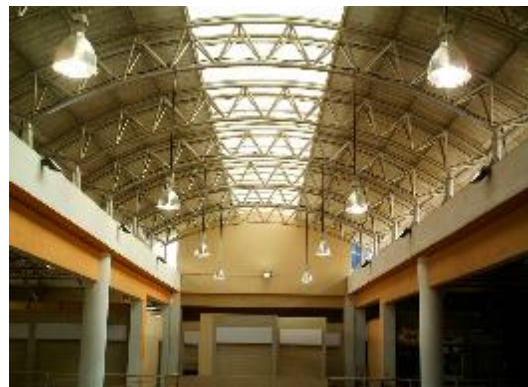
The lighting and the structure
